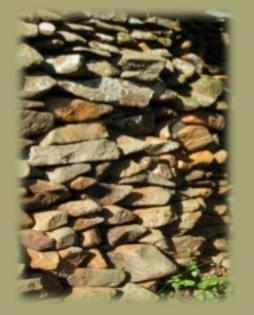
There is no mortar or cement between the stones to hold them together, yet the walls remain standing nearly 500 years after they were first built!
